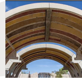
Dome roofing to keep sun out and effective for natural cooling
