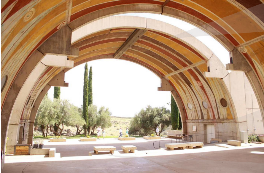
In the summer, the sun does not enter into the domed area
