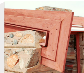
Stone structure supported by steel redwood beams
