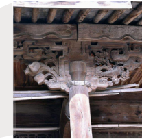
Wood structure for the old Mosque
