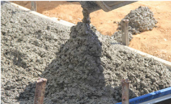
Fibercon concrete reinforced with recycled plastic as sidewalk
