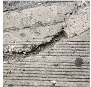
cracked pavement
