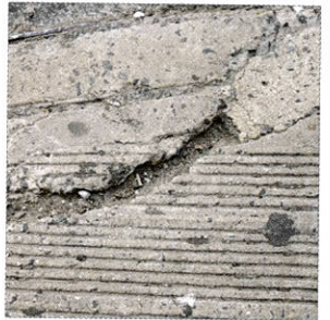
cracked pavement
